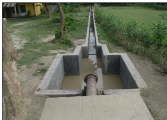
Figure 6: Deep Tube Well Operating System and Discharge Box
