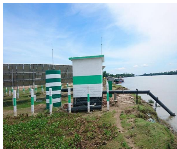
Figure 9: 5 Cusec capacities LLP in Sunamganj Sadar Upazila, Sunamganj.
