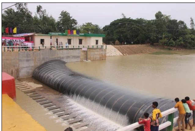
Figure 10: Chellakhali Rubber Dam, Nalitabari, Sherpur.
