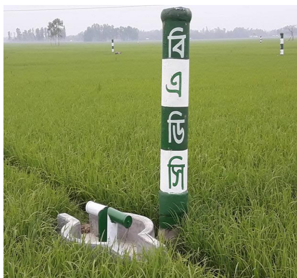
Figure 5: Electrically Operated Deep Tube Well and Buried Pipe Line.
