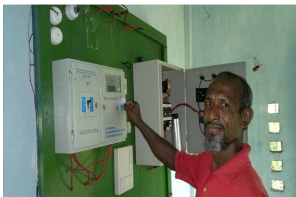
Figure 6: Deep Tube Well Operating System and Discharge Box
